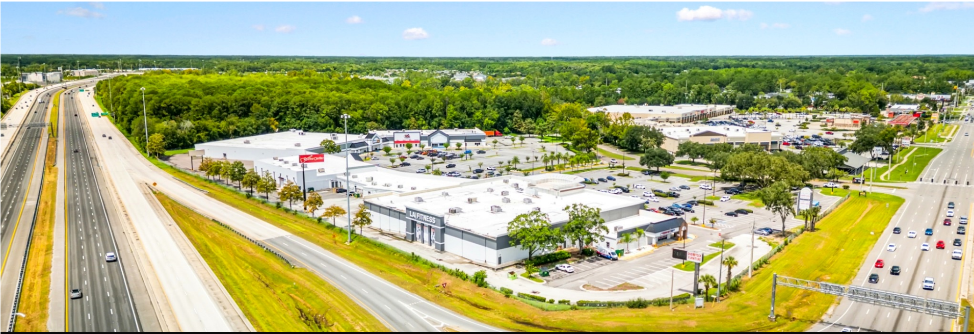
I-295 INTERCHANGE ACCESS
