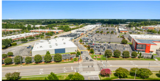
NORTH MALL ROAD CORRIDOR
