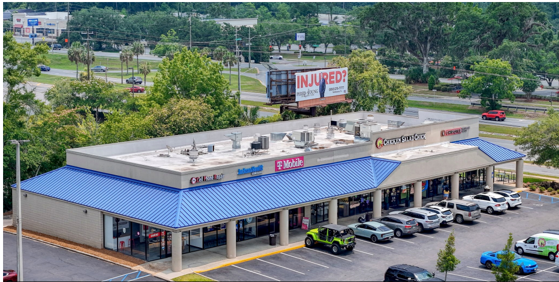
INLINE RETAIL FRONTAGE
